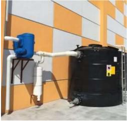
PFA RHS system is specially designed for urban rainwater harvesting.
